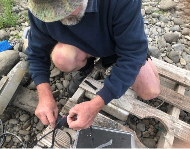
Repairing the raft for the HydroBoost product
